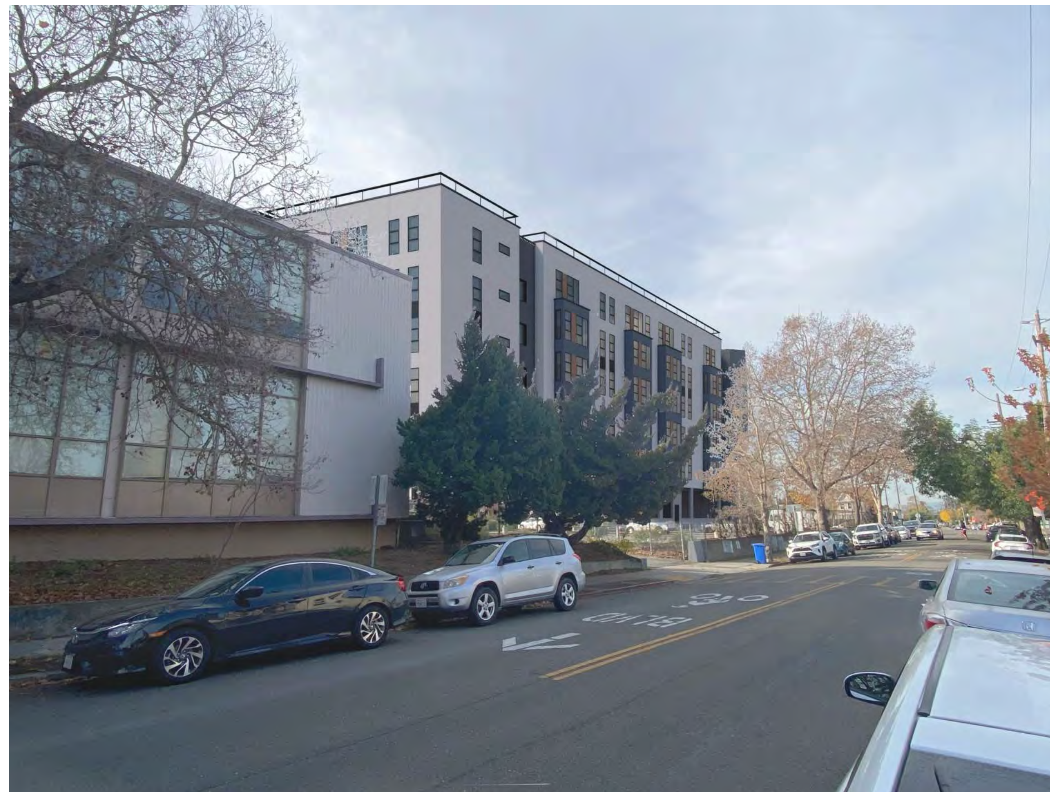
2. VIRGINIA ST. LOOKING WEST - AFTER
